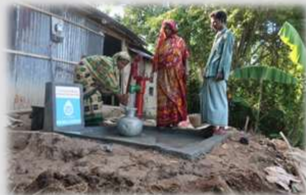
Photo: After the installation of tube well.
